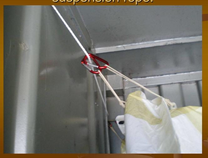
As you secure the ceiling ties, locate and secure the floor ties in the same method. NOTE: It is important the liner can fully extend once the clips are secured.
