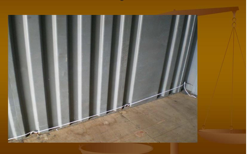
Locate the front top corner of the liner and secure the clips to the containers front top lash rings.
